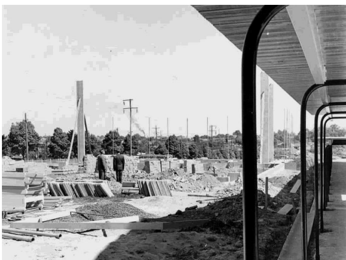
School Hall under construction. 1961.
