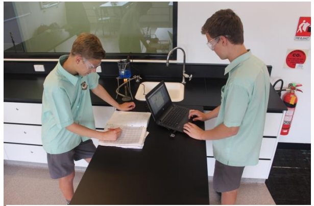
Extra power outlets cater for the use of data loggers and laptops
