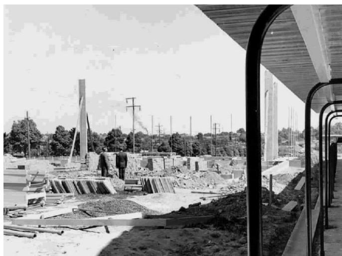
School Hall under construction. 1961.
